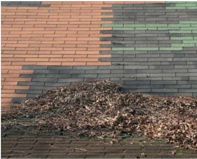
Sweet T. Pettway's roof, Gee's Bend
